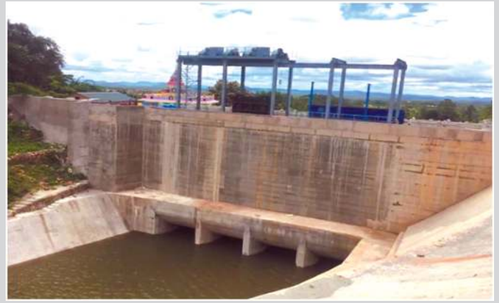
Head Regulator provided at Bhadra reservoir for lifting 29.90 TMC (UBP Package-2)
