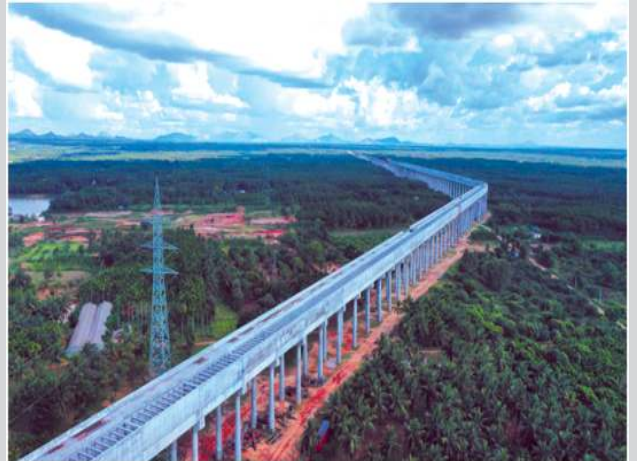
Major Aqueduct under Yettinahole Gravity Canal
