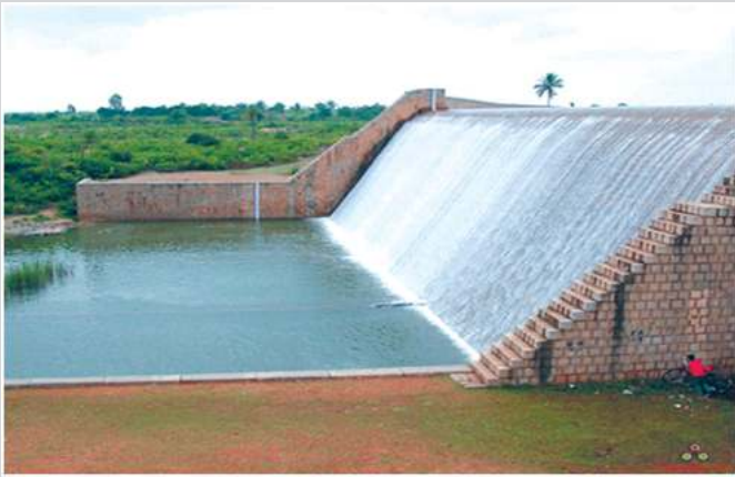
Stilling Basin of Gayathri Dam
