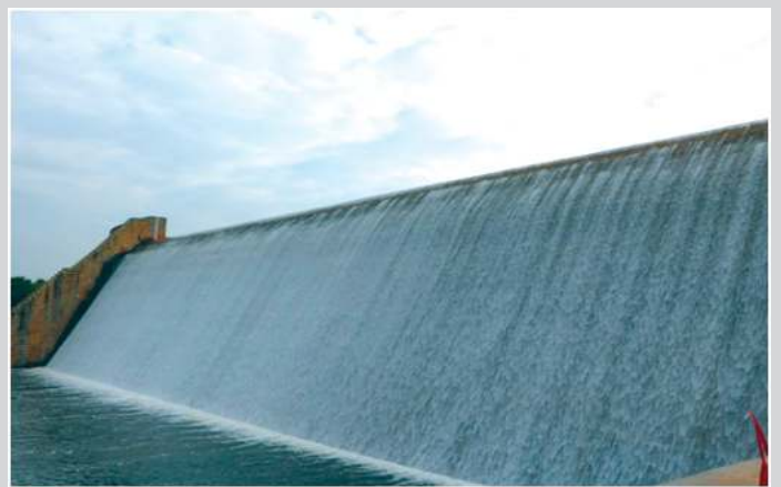
Spill way of Gayathri Dam
