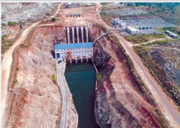
PUMP HOUSE-2 OF UBP PACKAGE-2
