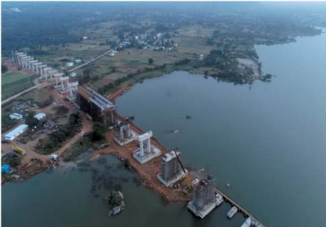
Aqueduct across Iraksandra tank under Yettinahole Gravity Canal
