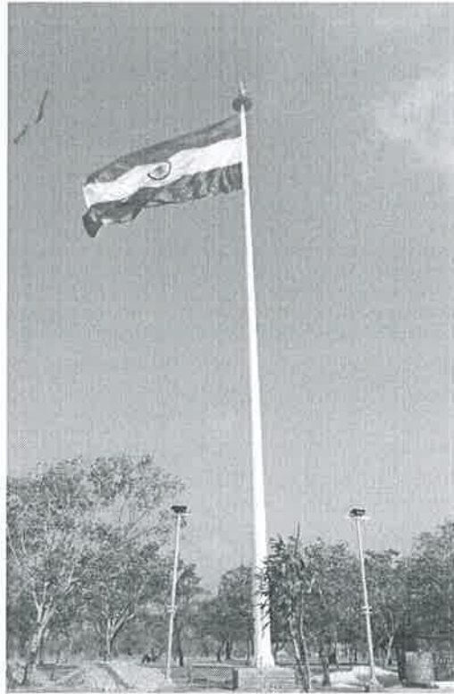
National flag (30.5 mts) mast and Park development work Near N.H.44
