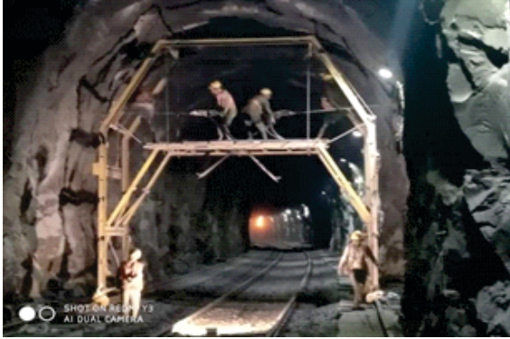
Rock bolting work at Ashti Tunnel
