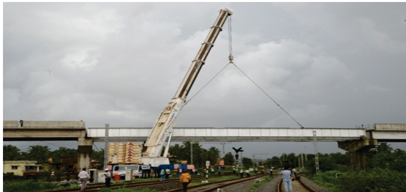
Launching of 45 meters length Steel Girders for Flyover near Thokur Railway Station
