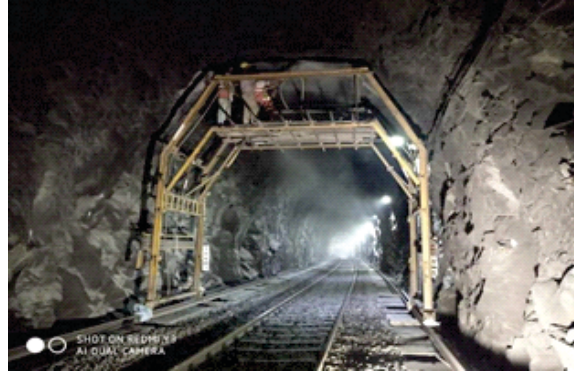
Shotcreting work at Ashti Tunnel
