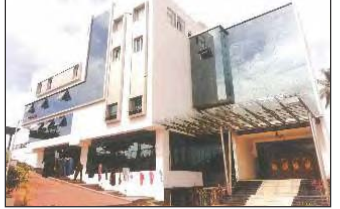
Commercial Complex at Hassan
