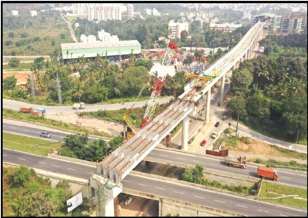
**Phase 2, Reach-4B - 53m Composite Steel Girder Erection across NICE Road**
