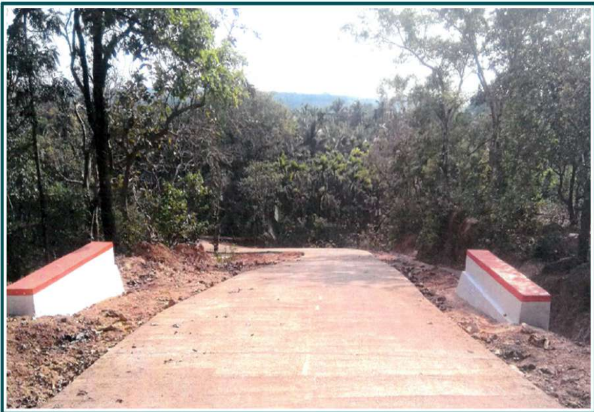
Pipe Culvert
