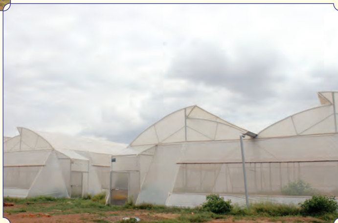
Shade House constructed at Main Campus UHS, Bagalkot during the year 2017-18
