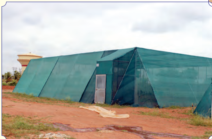
Green House constructed at Main Campus UHS, Bagalkot during the year 2017-18
