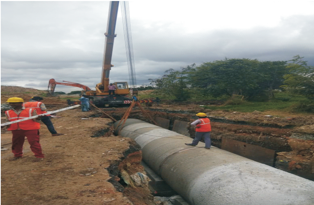
CE WWM 2017-18 Work of Pumping main from Koramangala sports complex ISPS to K & C Vally STP under AMRUT – Package S2D(a)
