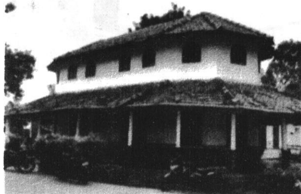
Inspection Bungalow ,Dambala
