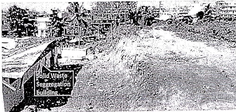
Photo 6(a) – Bund of Gowdanapalya tank cut and width diminished to accommodate a building for Solid waste segregation and further to accommodate Storm Water Drain
