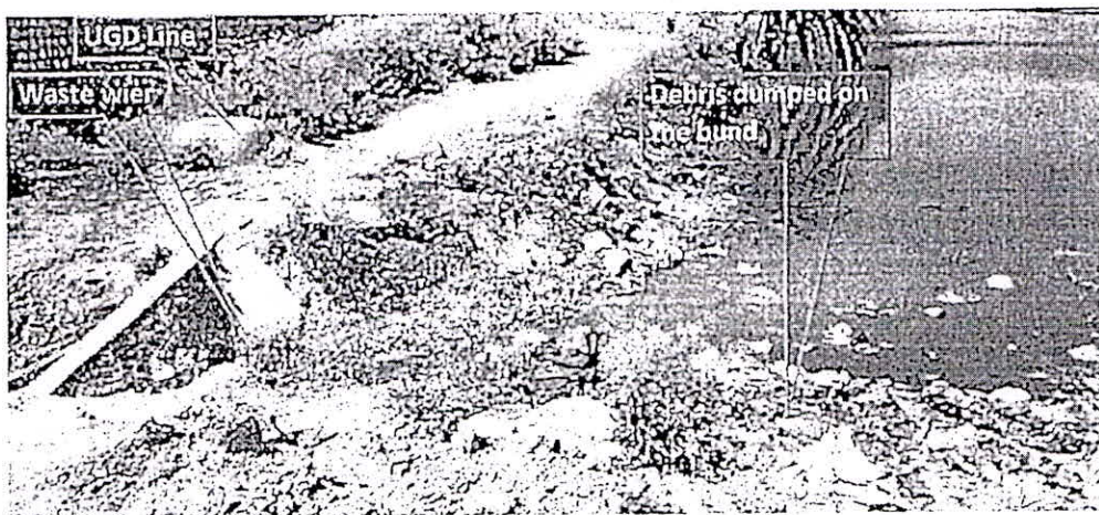
Photo 7(a) above & 7(b) below – Waste weir of Kelaginakere Bairasandra tank is completely encroached with debris. UGD lines are carried in the tank bund. Tank bund is encroached by filling the debris. Storm water drain is being constructed by the side of compound wall.
