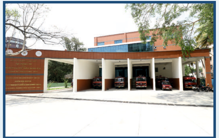
Construction of 6 Bay Fire Station at Mayo Hall in Bengaluru
