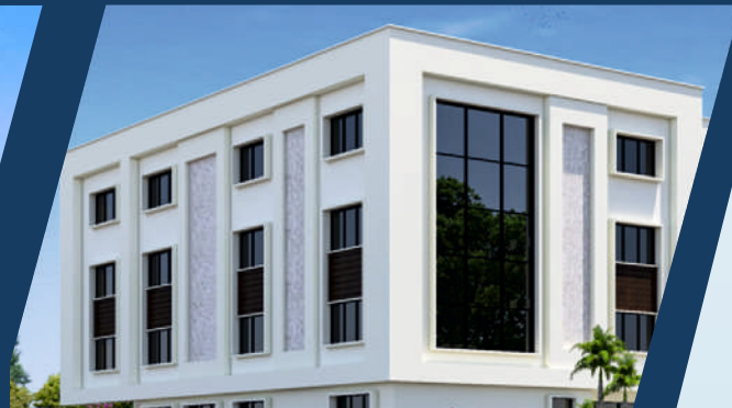
Construction of Highgrounds Police Station & Traffic Police Station & Seshadripura ACP office
