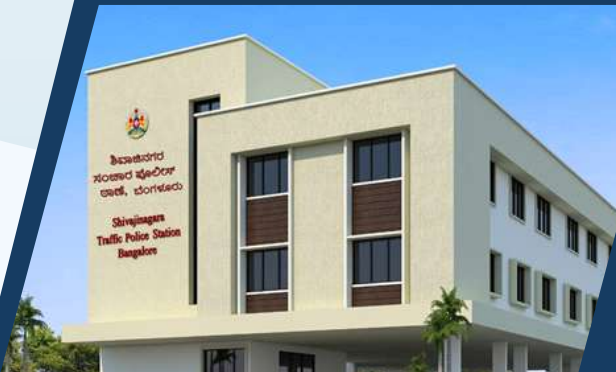
Construction of Traffic Police Station at Shivajinagara
