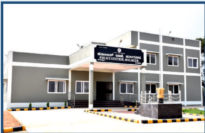
Construction of Police Station at Hulagur in Haveri Dist.
