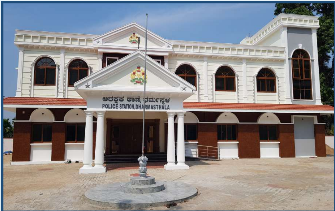
Construction of Dharmasthala Police Station, in Dakshina Kannada Dist.
