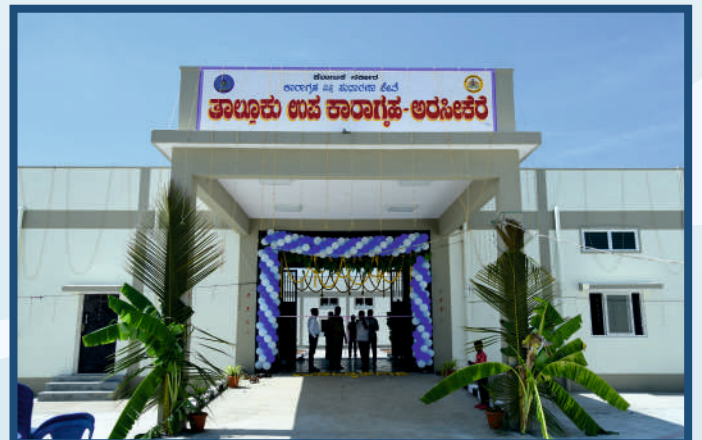
Construction of Sub-Jail at Arasikere, Hassan District
