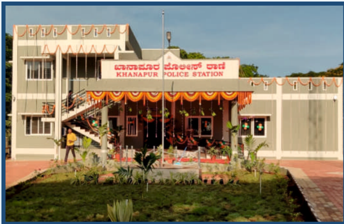
Construction of Khanapur Police Station in Belagavi Dist.
