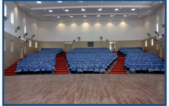
Construction of Multipurpose Auditorium & 60 Nos capacity Classroom in 1st floor for PTS at Dharwad
