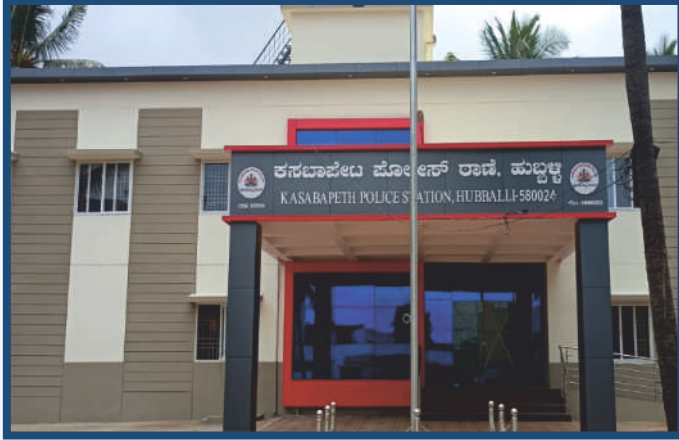
Construction of Kasabapeth Police Station in Hubballi Dist.
