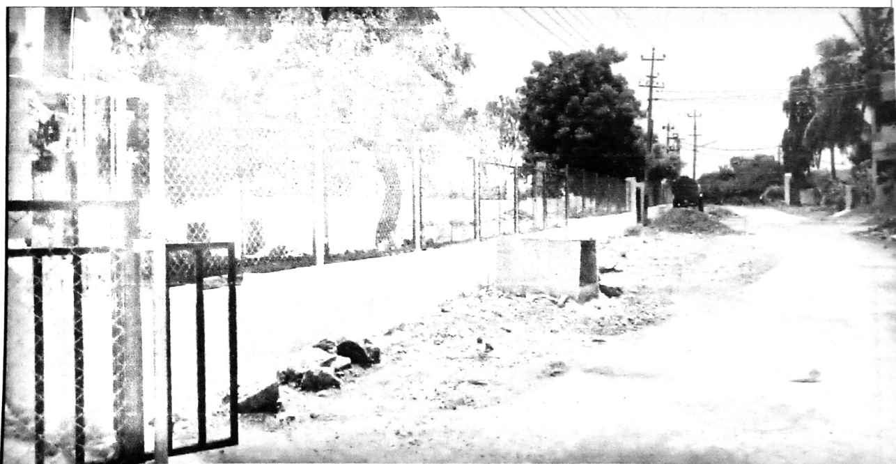
SL.No-2 Providing And Fixing Compound Wall With Fencing Work At Siddeshwar Gadagi Layout Near Shri.Jai Hanuman
