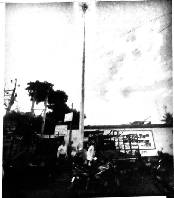
S.L-27 Construction Of 16 Mtr High Mast Pole At W.No.16 Gandhi Nagar Near Star Chowk.
