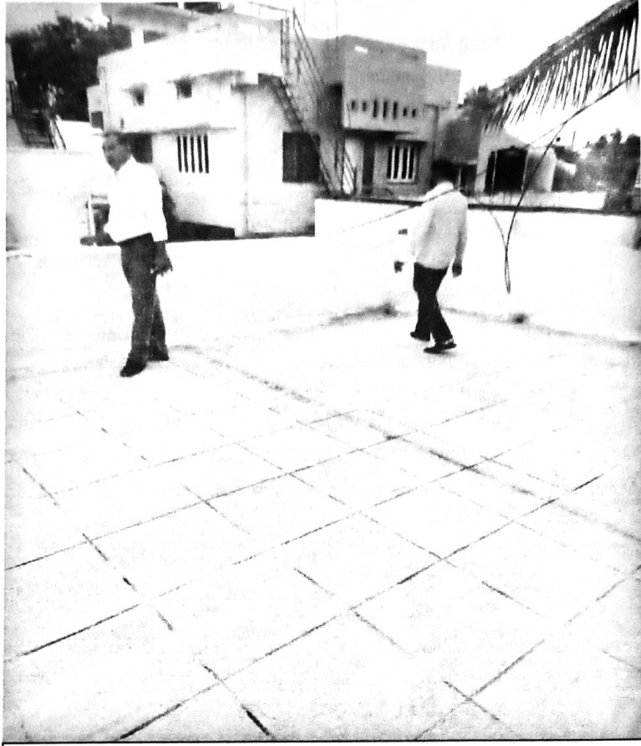
S.L.31 Repairing, Painting & Water Proofing At VUDA Commissioner, AE & Office Staffs Quatars.
