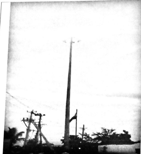
S.L-27 Construction Of 16 Mtr High Mast Pole At Gachinakatti Colony Near Bali Parshi Adda.
