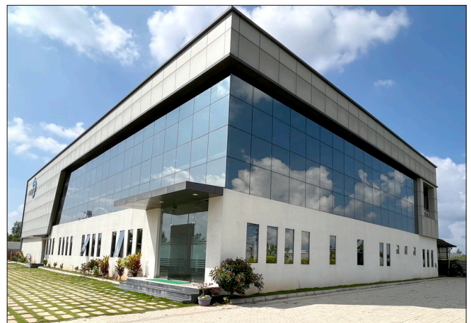
Automation Unit in Bengaluru Rural Dist.
