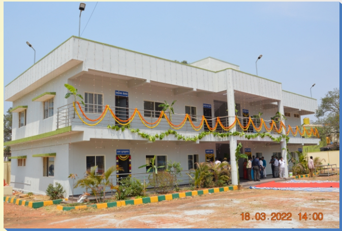
New Bus Depot at Devanahalli
